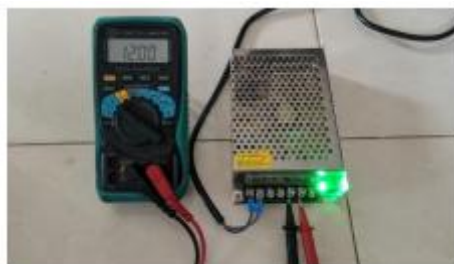
Figure 18. Power Supply Testing
